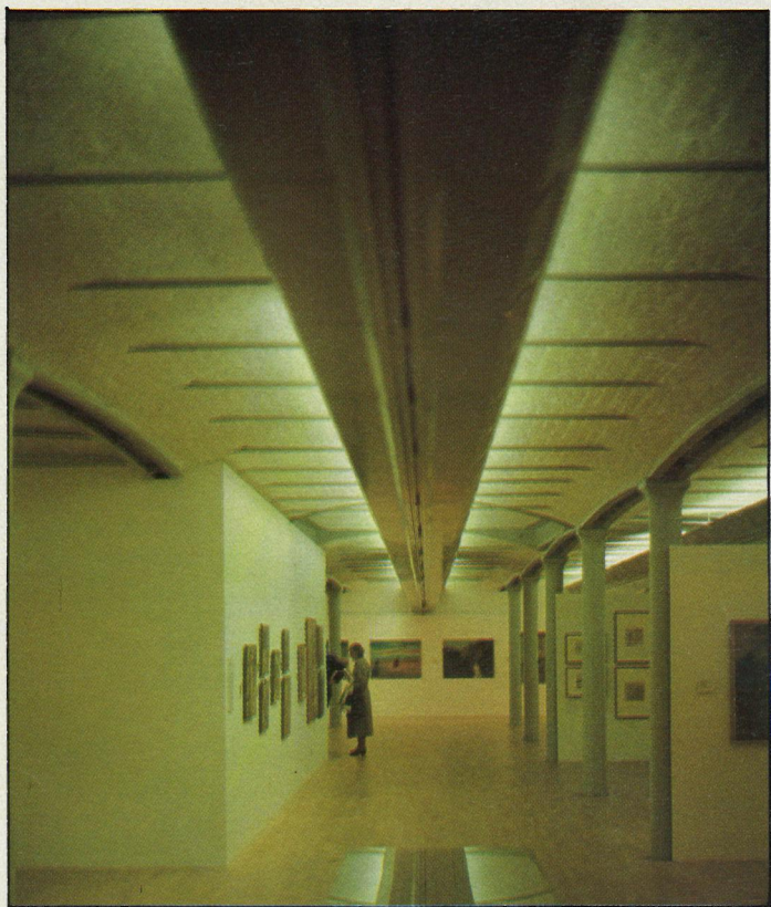
A view of one of the services booms carrying lighting, air conditioning, smoke detectors and loud speakers on the first floor of the Liverpool Tate.
